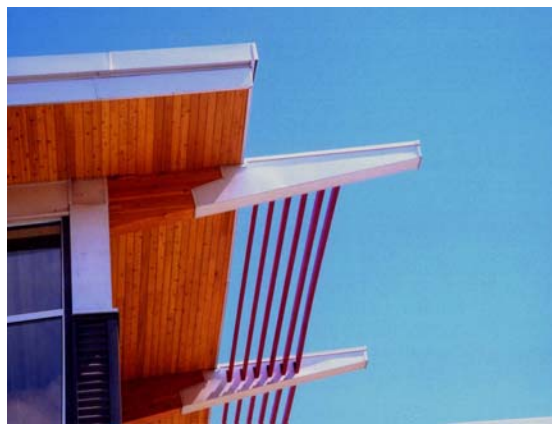
Figure 2. Cap flashings at exterior truss extensions
