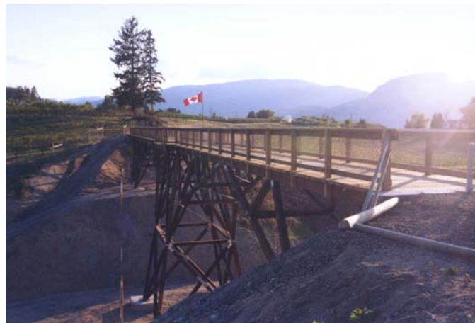
Figure 9. McCulloch Trestle, Kettle Valley Railway, BC
