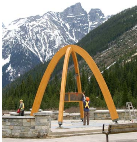
Figure 7. Replacement arches at Roger's Pass, BC
