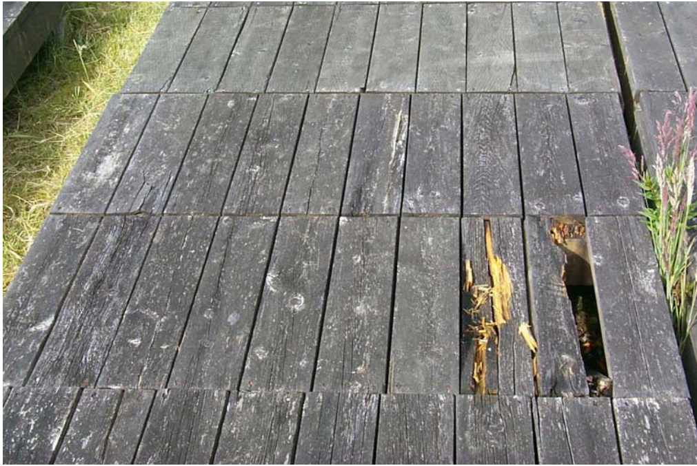
Figure 3: Lodgepole pine untreated deck in Vancouver
