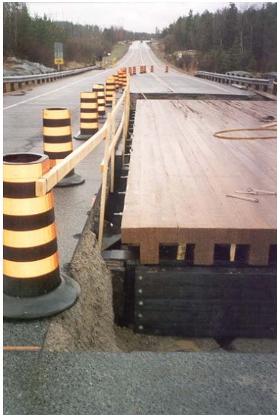
Figure 2 SCL Tee Beams under construction at Rushing R.
