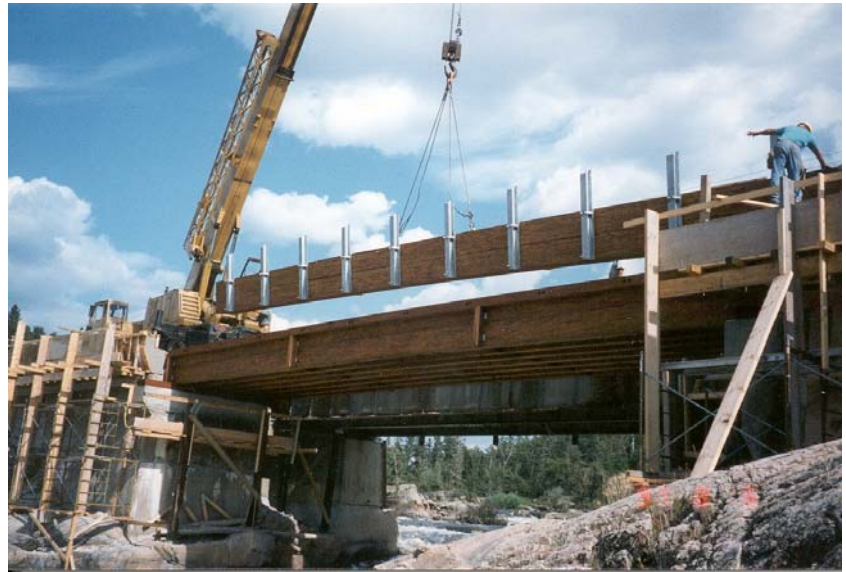
Figure 3 SCL Tee Beams under construction at Wabigoon R.
