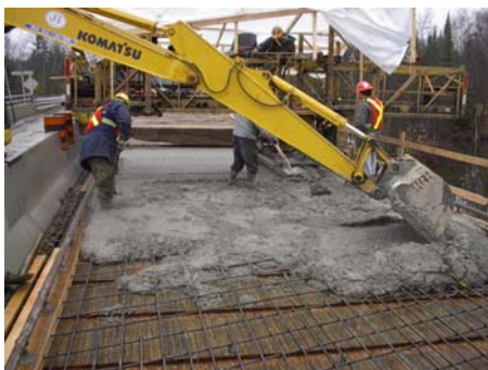
Figure 4 SCL/Concrete Composite construction at Blind R.
