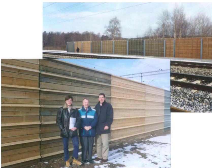
Figure 11. Noise barrier of larch with test sections of pine ( Pinus sylvestris ) treated with different arsenic and chromium free wood preservatives. Test sections with untreated spruce ( Picea abies ) and pine ( P. sylvestris ) are also included in the trial.
