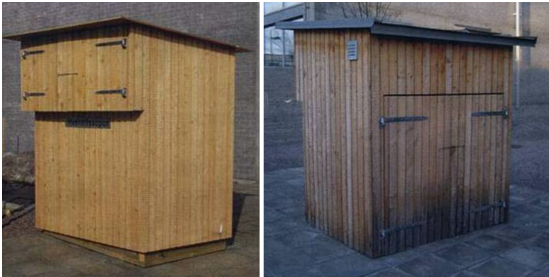
Photo 8: Untreated larch heartwood structure
