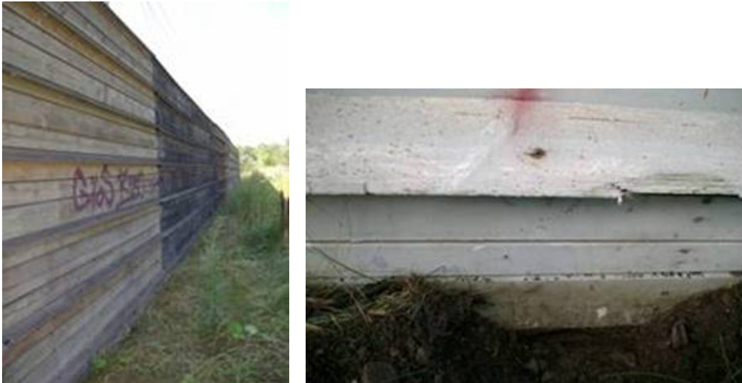
Photo 3: Noise barrier near Stockholm Sweden after 8 years in service (ScanImp treatment)
