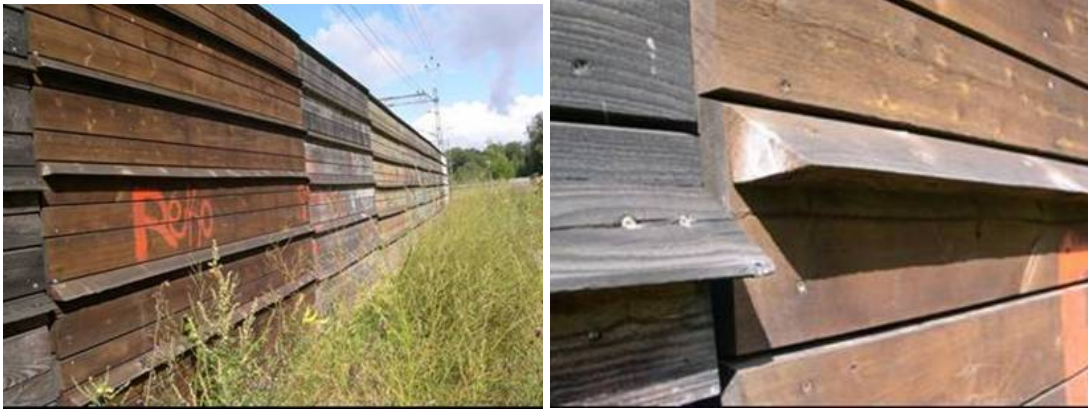
Photo 2: Noise barrier near Stockholm Sweden after 8 years in service (Royale treatment)
