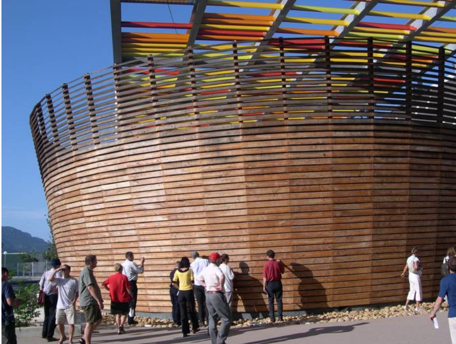
Photo 7: Thermal heat treated structure, Montpellier France
