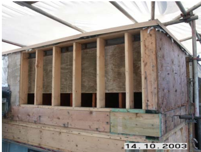
Photograph 5: Replaced wood framing. Treated wood is visible.
