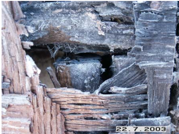
Photograph 3: Decayed plywood.
