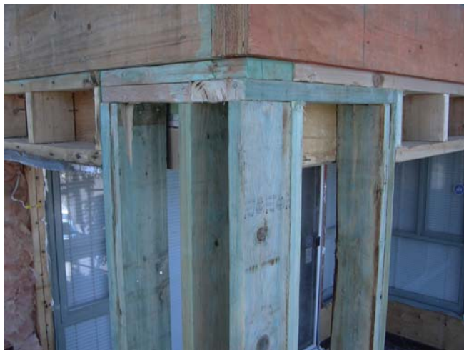
Photograph 6: New wood framing at the balcony column.
