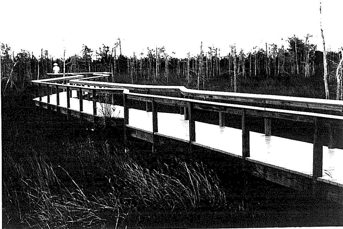
Figure 3 Wood-supported recycled-plastic-lumber walkway
