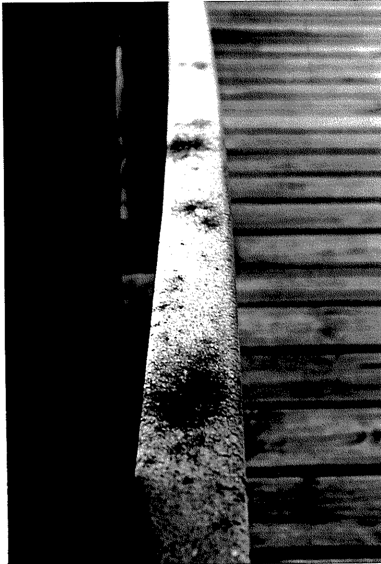
Figure 7 Bluestain on the surface of plastic/wood composite lumber
