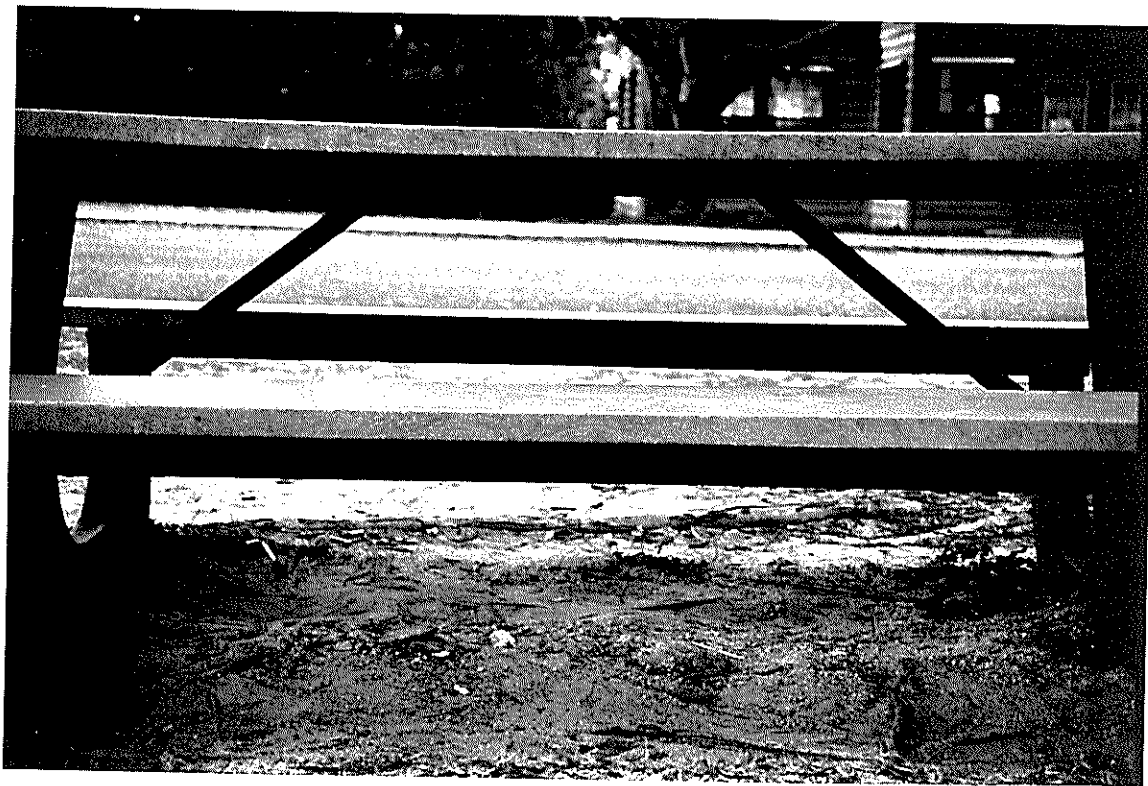
Figure 2 Metal-supported recycled-plastic-lumber picnic table
