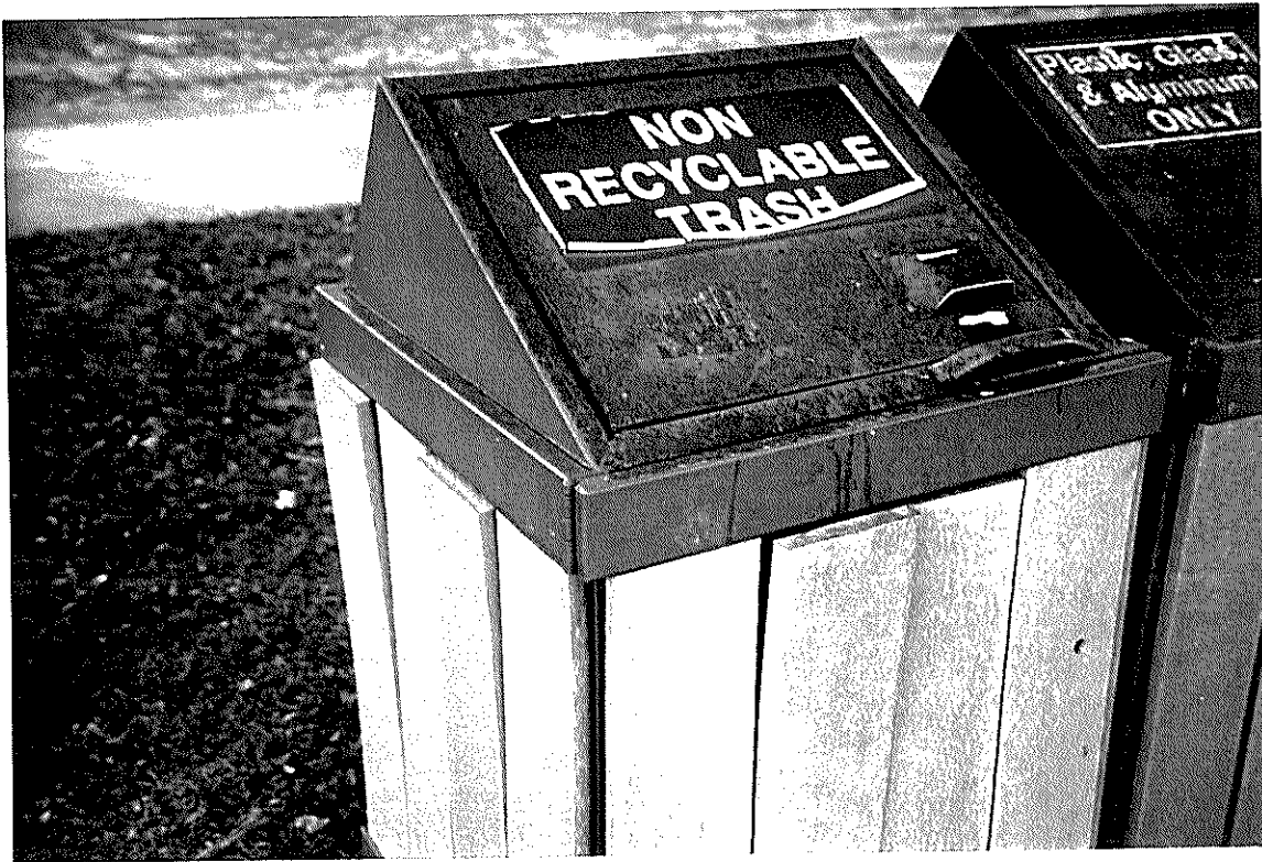
Figure 9 Trash container showing warping of recycled plastic lumber
