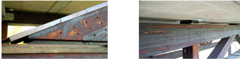
Figure 1 Kjøllesæter hybrid timber bridge in Rena with a concrete deck
