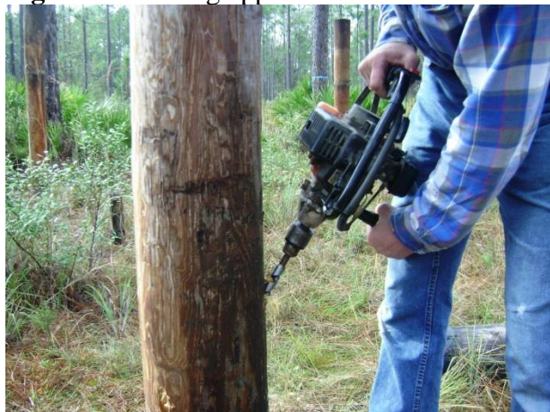
Figure 1. Drilling application holes.
