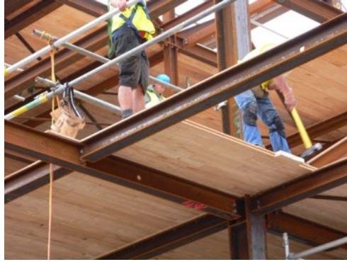
Figure 3 - A hybrid structure consisting of steel frame and wood floor panels.
