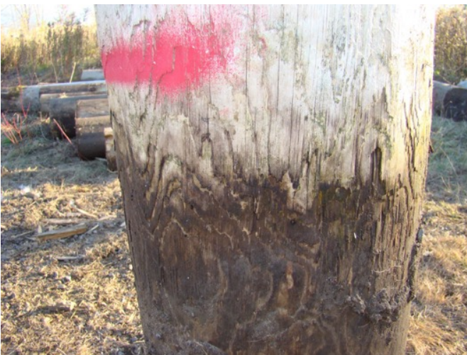
Figure 6: Pole section remediated with Pole Wrap after 11 years in the ground
