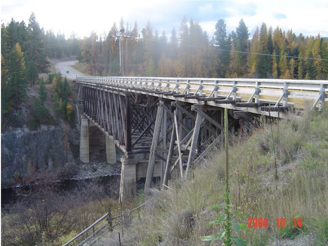
Figure 1 – The St. Mary's Wycliffe Bridge, built in 1931, illustrates the durability of some timber structures, the lack of redundancy in long span trusses, the difficulty of replacing deteriorated truss members and thus the importance of good preservative treatment.
