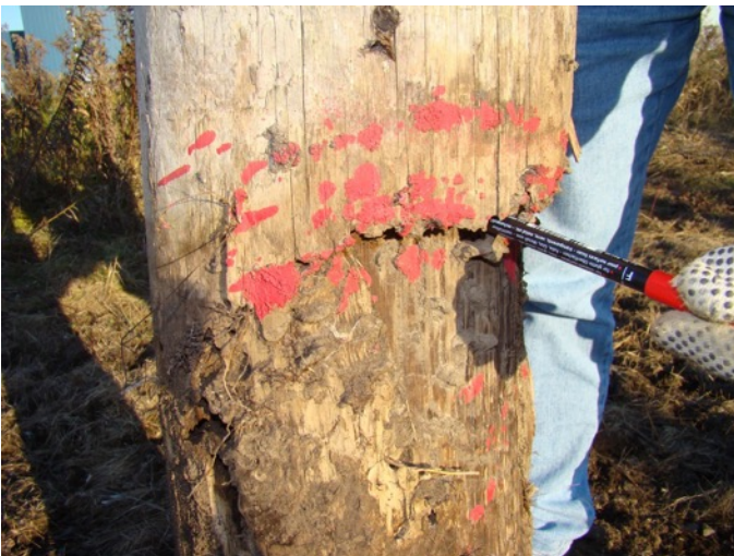
Figure 4: Ground line section for a jack pine reference after 11 years in the ground
