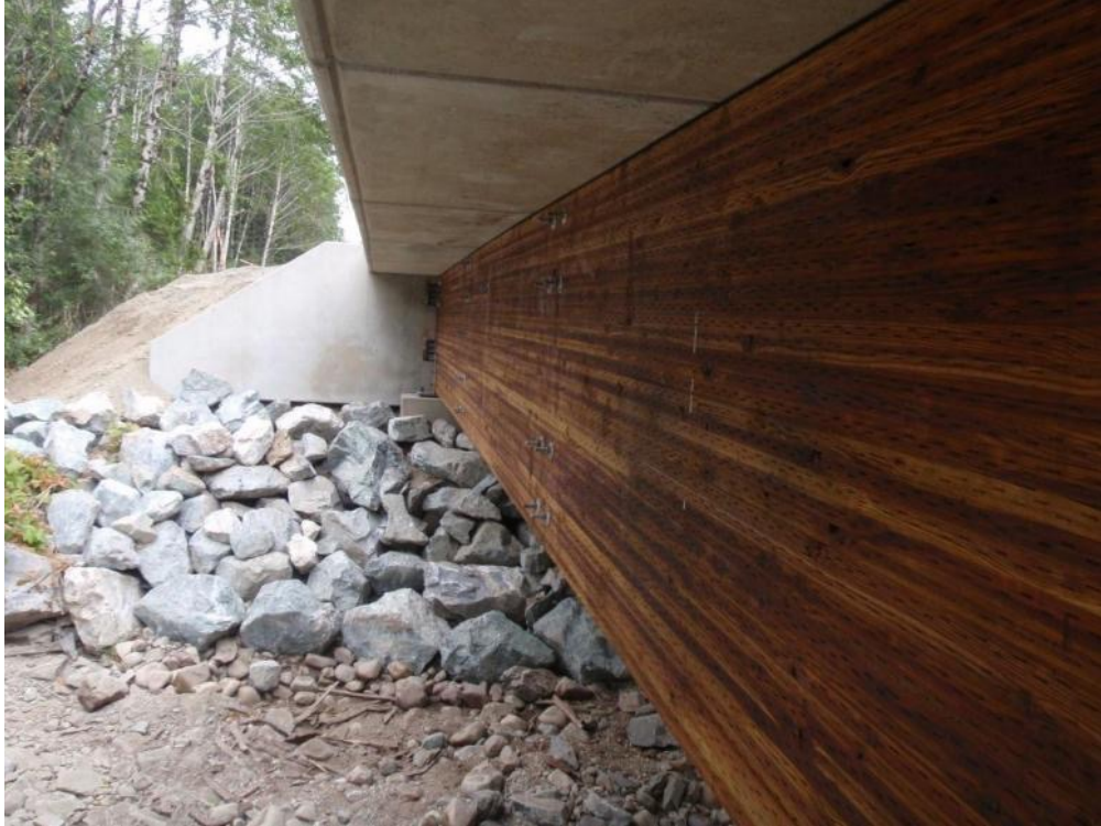
Figure 2. The Large Creek Bridge, built in 2010, has glulam girders with a concrete deck and foundations.
