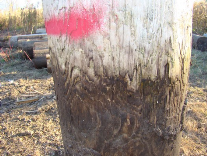
Figure 5: Pole section remediated with cobrarods after 11 years in ground.
