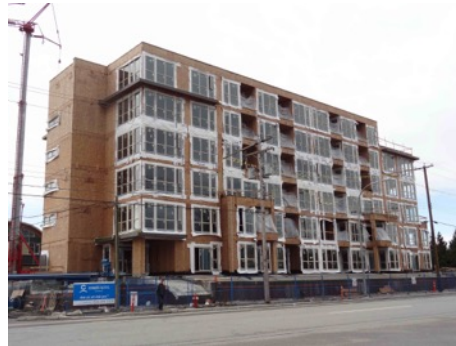
Figure 2 - First 6-storey light wood frame building in BC.
