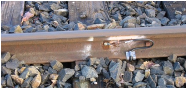
Figure 1. Signal connection on ACZA Douglas fir tie
