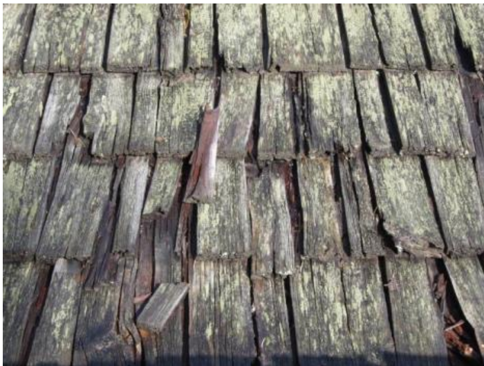
Figure 6 Untreated pine shakes at Vancouver after 15 years.
