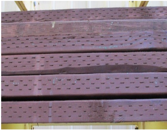
Photo 1: Incised Douglas fir pre-stained to intended to resemble redwood and then treated with copper azole
