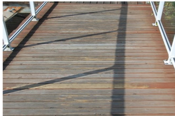
Photo 4: Pre-stain decking showing track wear patterns from foot traffic.
