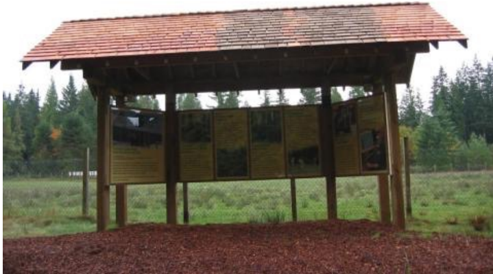
Figure 2 Sign shelter from the north immediately after installation at Maple Ridge.
