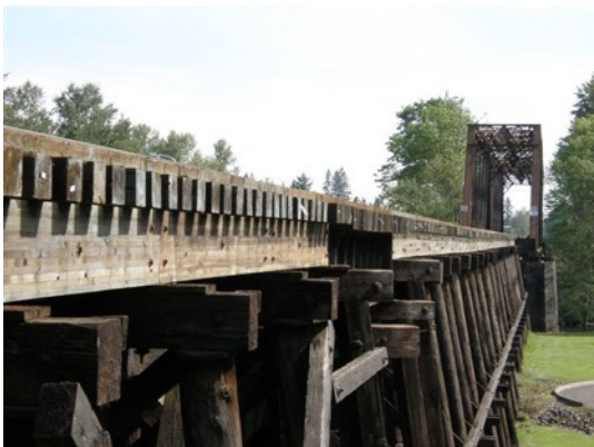
Figure 10. ACZA Douglas fir ties on a bridge trestle over a stream
