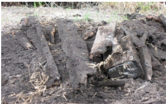
Seven Year Old Ties being removed
