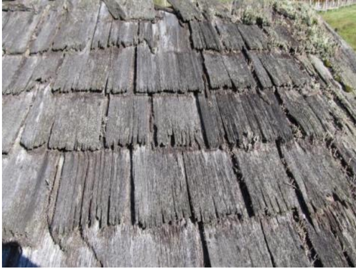
Figure 3 Untreated western redcedar shakes at Maple Ridge after 40 years
