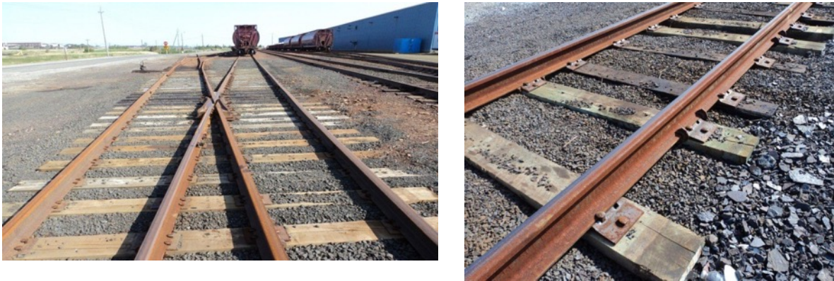
Figure 9. Canadian ACZA Hardwood Tie Installation
