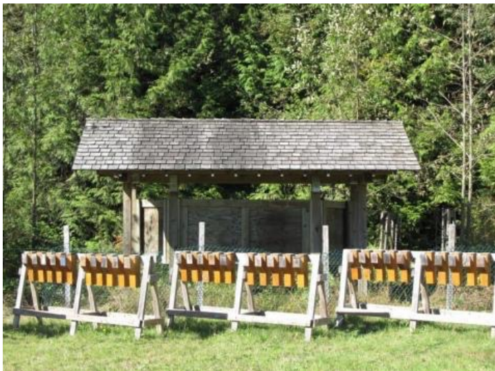
Figure 7 Sign shelter from the south after 10 years in test ( \gamma -joint test of field cut preservatives in foreground)
