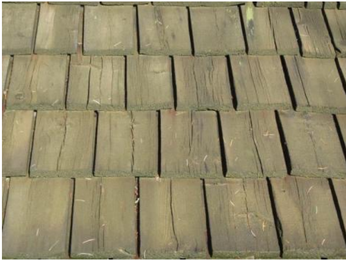
Figure 5 CCA-C-treated pine shakes at Vancouver after 15 years.
