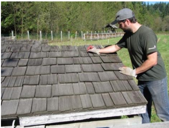
Figure 4 Inspection of CCA-B-treated western redcedar shakes at Maple Ridge after 40 years
