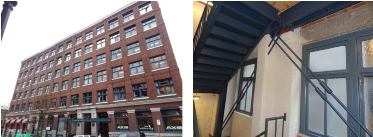
Figure 8: Leckie Building and seismic reinforcement
