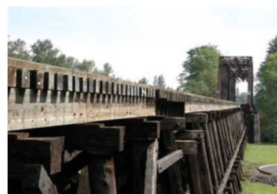
Bridge Ties and Laminated Beams
