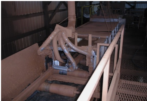
Photo 3: Typical configuration of pre-stain spraying equipment.
