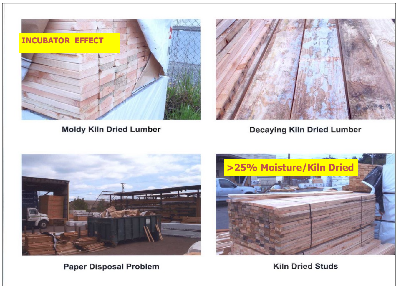
Figure 5. Improperly dried and improperly stored lumber showing mold/stain/decay development.
