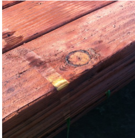
Photo 9: Colour variation associated with tight banding and corner protectors
