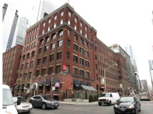
204-214 King Street East Built 1901 - 7 storey – 134,430 ft 2
