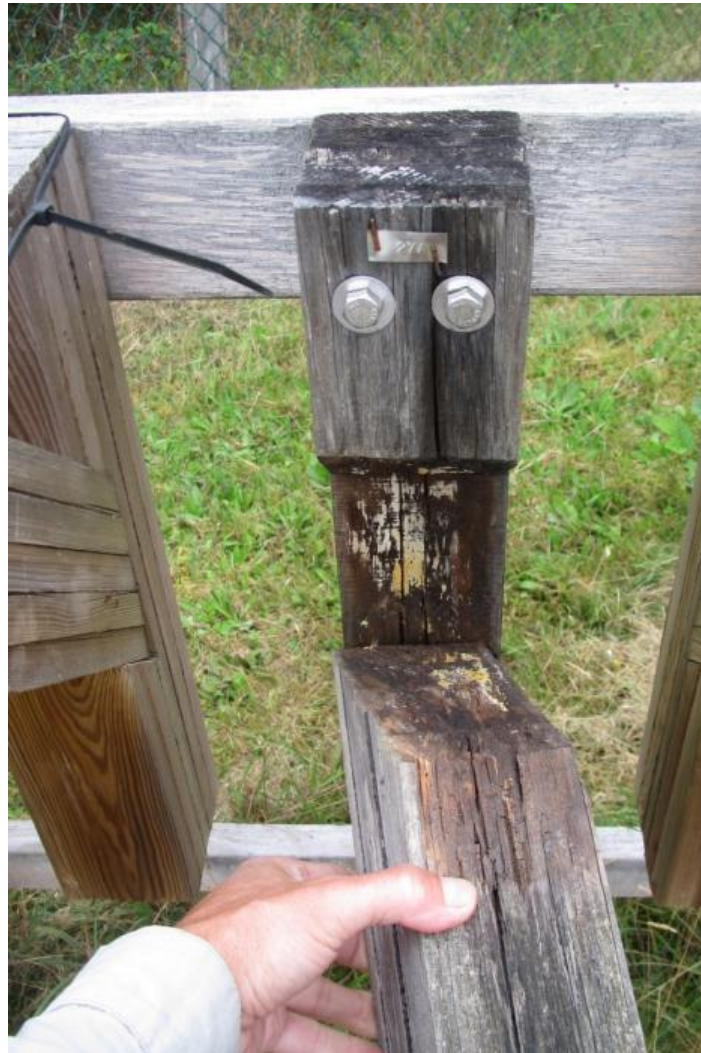
Figure 8 Decay after six years in untreated glulam \gamma -joint installed above ground
