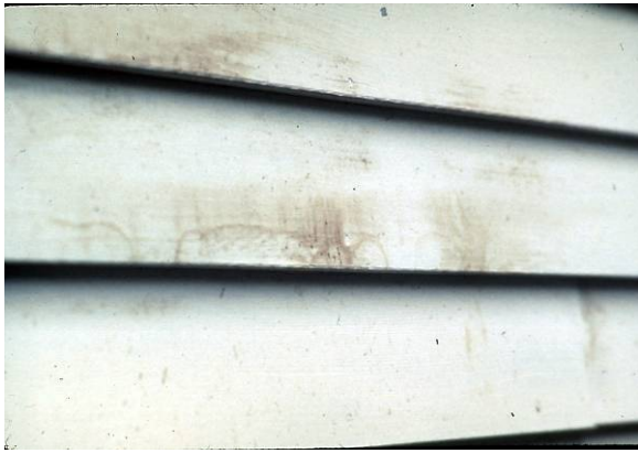
Figure 13. Diffuse extractives bleed on painted boards
