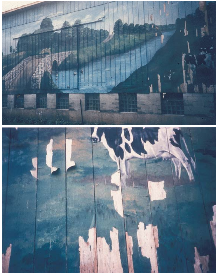
Figure 16. Mural on barn near Madison, Wisconsin (top); close-up of paint failure (bottom)
