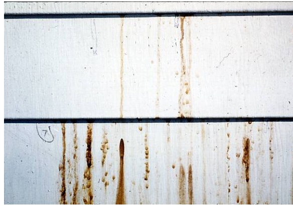
Figure 14. Run-down extractives bleed on painted boards
