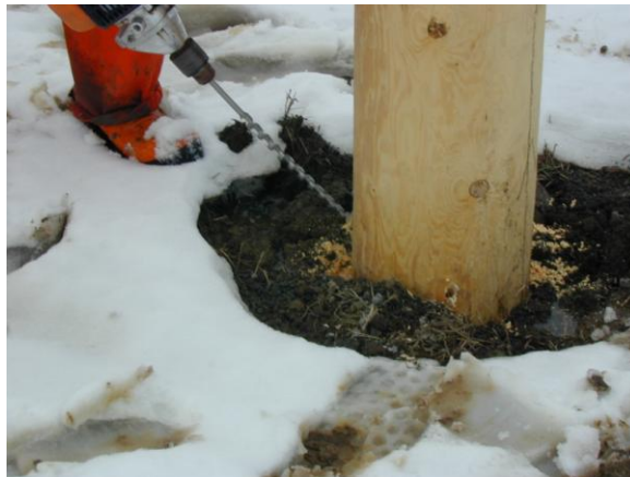
Figure 3: Drilling of the pole section to insert the rods
