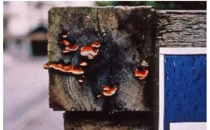
Figure 5 Cut Ends Without Field-cut Preservative Decaying in 8 Years in Whistler BC
