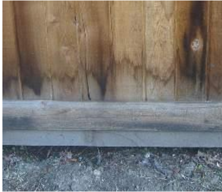
Figure 1. The Built-to-Rot Cedar Fence
