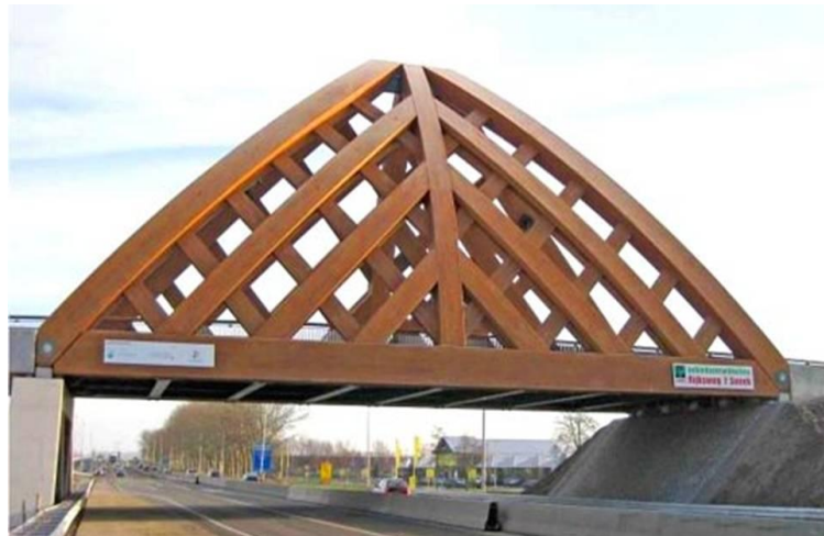
Figure 5 - 60 Ton Bridge, Sneek, Netherlands
