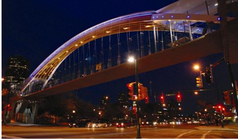
Figure 6 - Kingsway Pedestrian Bridge, Burnaby, BC
