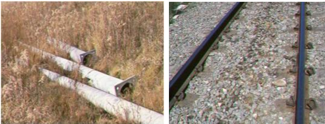
Figure 2: Examples of alternative materials – steel poles and concrete ties
