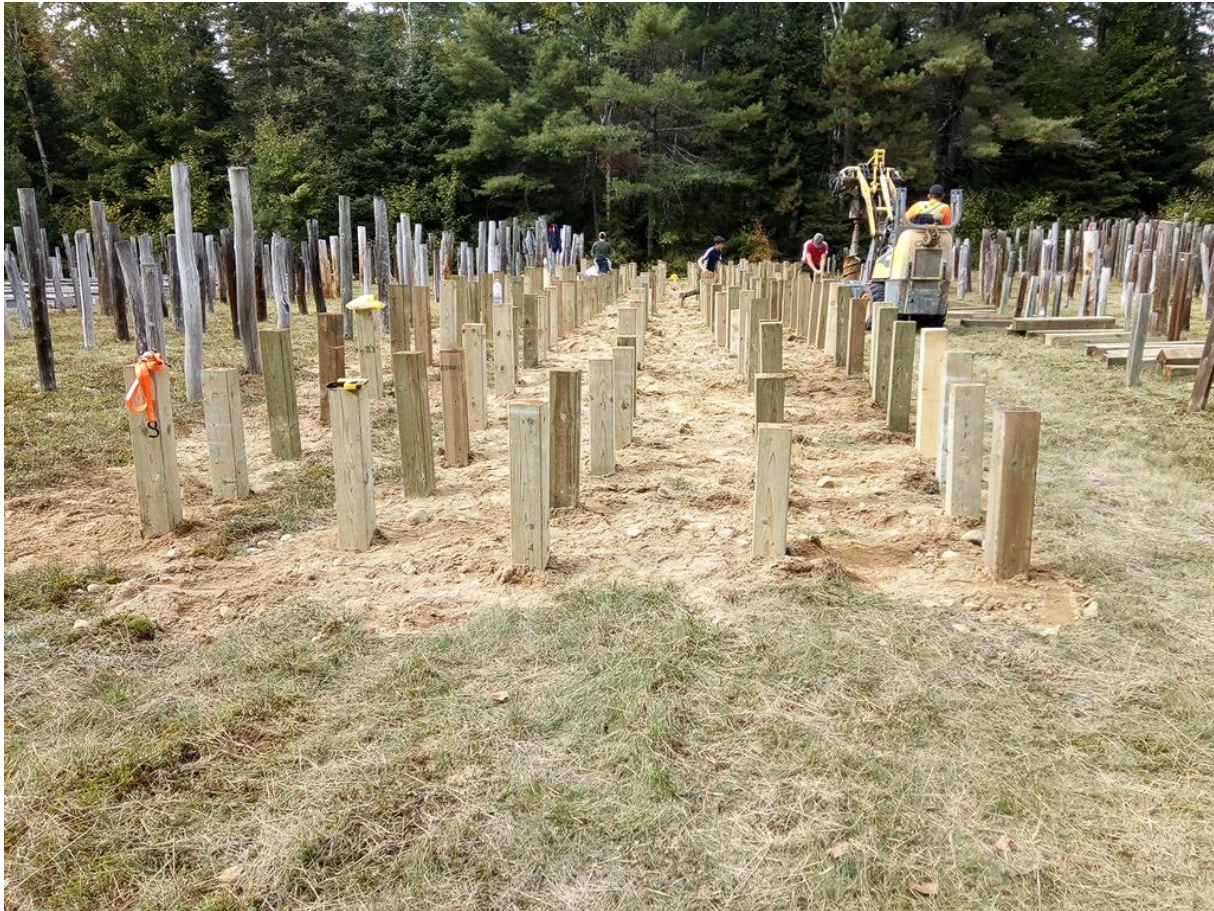
Figure 5.- Red Pine Posts being installed at the FP Innovations Test Site in Petawawa Ontario
