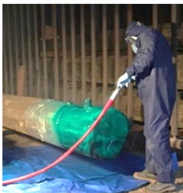
Figure 1. Application of polyurethane coating around sticks' end
